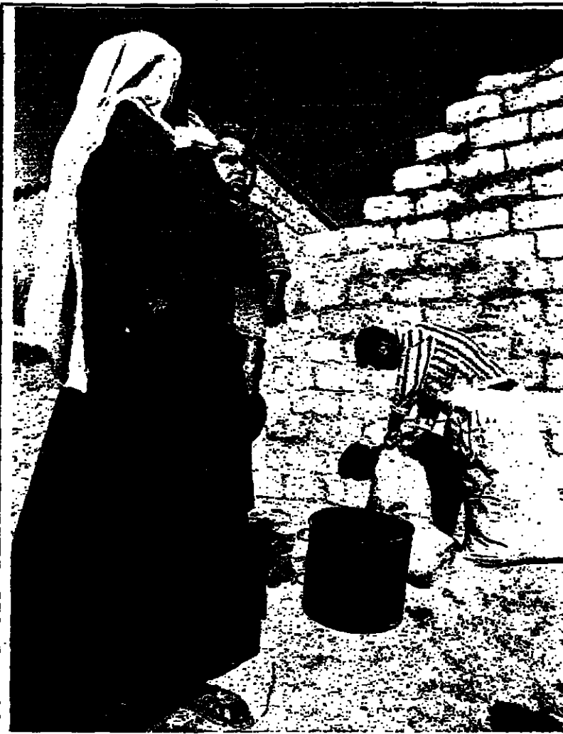
Resident of Rafah camp building additional room to his new dwelling outside the camp from bricks which he took from his former home, watched by his wife. Families whose homes are being demolished for wide roadways have been given housing near the camps on easy terms — and many quickly collected bricks and other material from their old homes to add to their new houses. (Bar-Tal)
